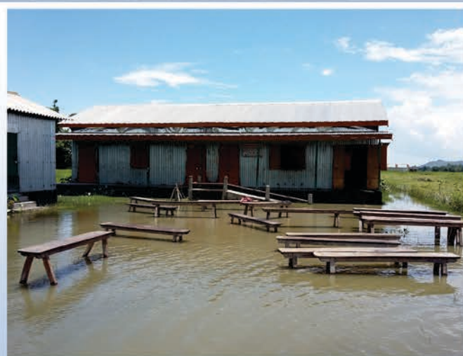
Flood water inundated the school premise
