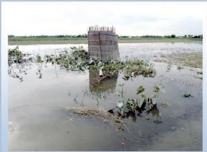
Condition of a kuccha toilet in char area after the flood
