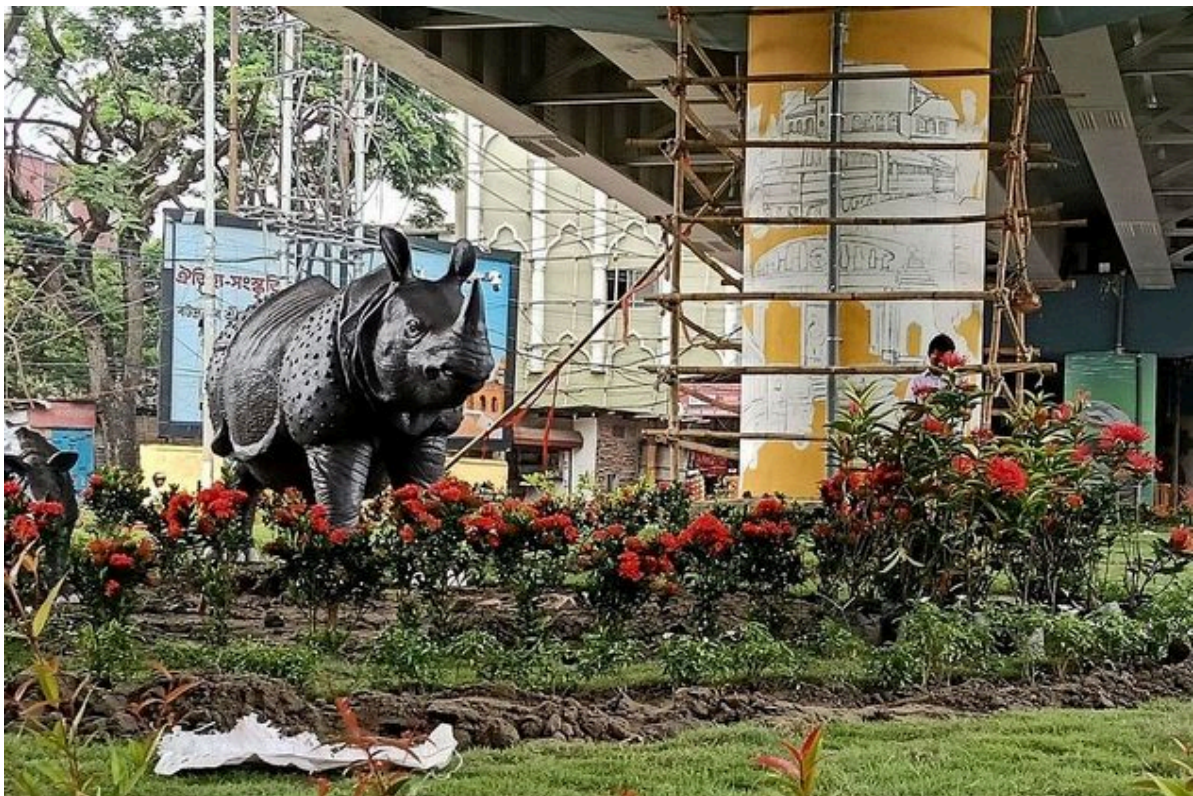
Workers carry out beautification work near Guwahati Club Rotary in Guwahati on June 23, 2026, as the city underwent extensive preparations ahead of the proposed India-Japan summit. Photo: UB Photos
